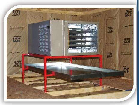
How would you install an attic system like this: cinder blocks & wood, a drain pan on 2x4's?
